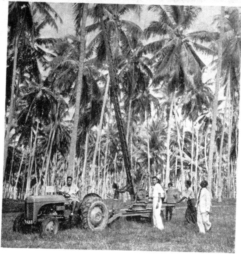
The Escalator Ladder.
