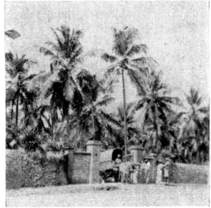
Main entrance, showing typical mud wall
