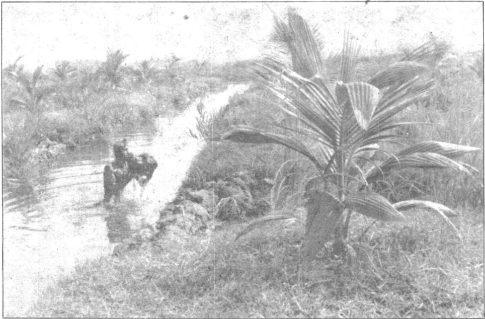
Filling of drains using soil excavated from the main drain.
