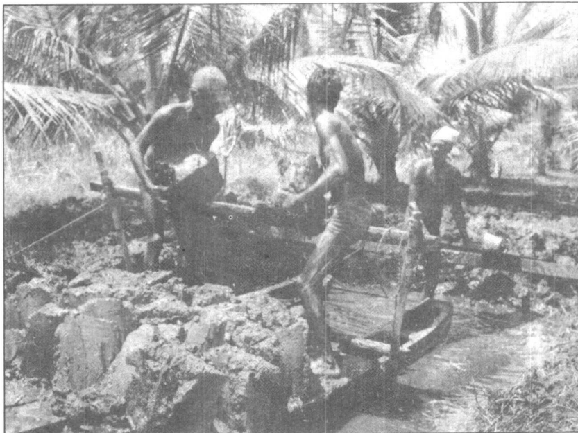
Filling the main drains with transported soil
