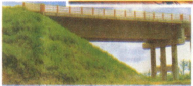
Grass being grown on an embankment after laying of Geotextiles
